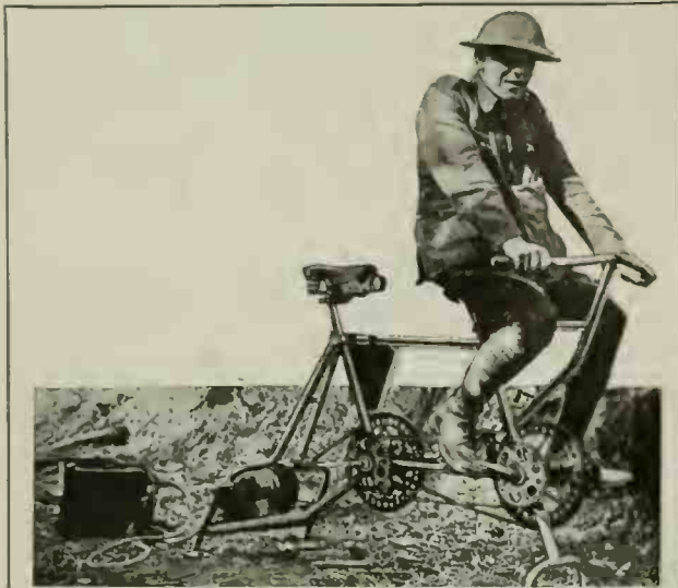
The Above Illustration Shows an Ingenious German Method of Generating Electricity for a Wireless Installation in the Trenches, Captured in a British Advance. A tandem bicycle with its wheels removed has been fitted with a supporting frame so as to stand upright and the pedal wheels connect with a belt to a small dynamo.
