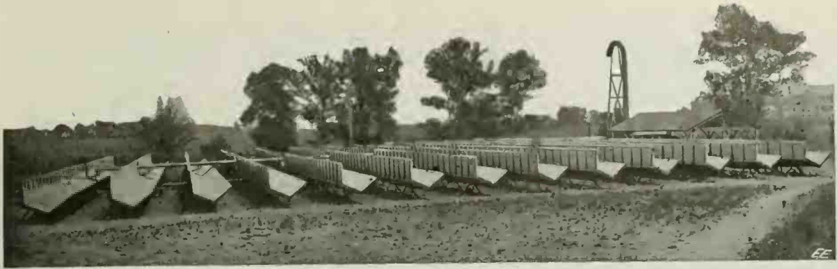
Some Day in the Near Future We Shall Undoubtedly See Hundreds of These Solar Energy Plants Sprinkled Over the Country. This Large Plant is in Texas. The Mirrors Reflect the Sun's Rays Onto Special Boilers, the Steam Produced Running a Steam Engine, Connected to a Dynamo. Current From the Dynamo Runs a Motor Pump Which Lifts Water to a Height of Sixty Feet.
