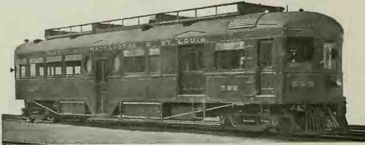
The Latest Type of Gas-Electric Car. It Is Driven by Electric Motors Which Derive Their Power from an Oil Engine Driven Dynamo. A Storage Battery Floats On the Electric System to Care for Extra Demands On Ascending Grades, Etc. No Trolley Is Required as the Power Plant Is Self-Contained. Electric Drive Is Used to Maintain Even Engine Speed and Great Flexibility of Drive.
