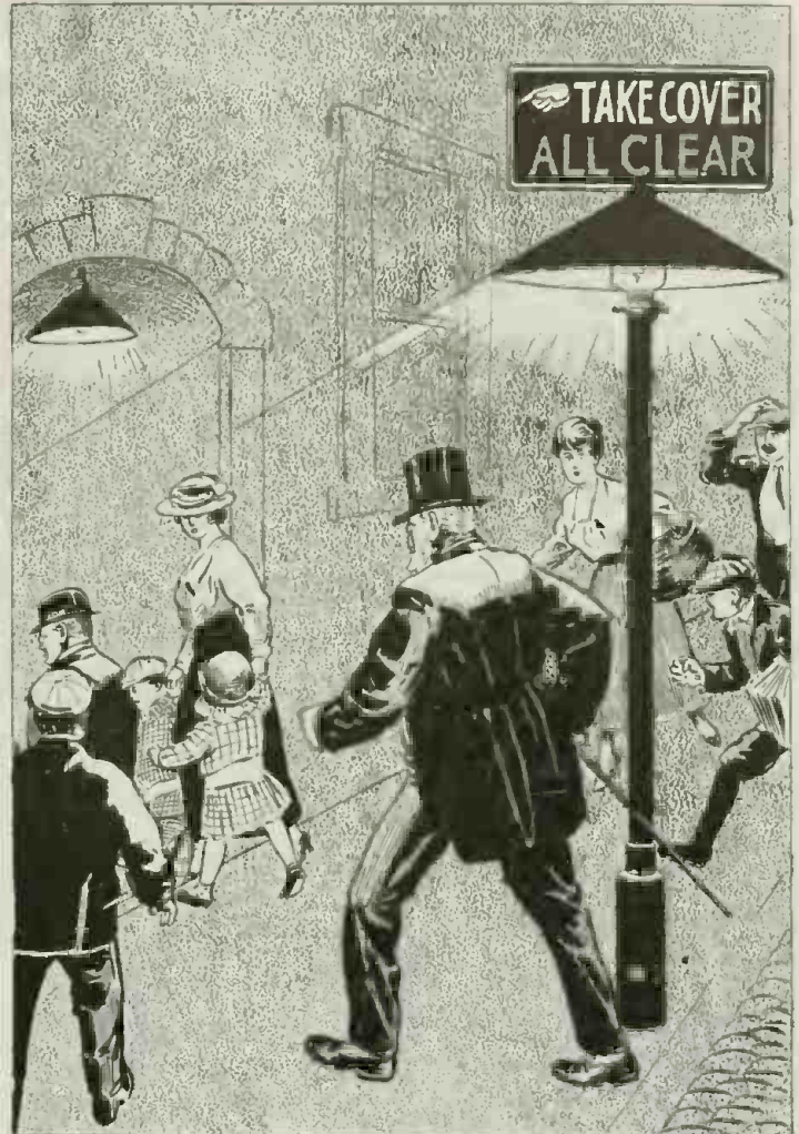
London and All the Larger English Cities Are Now Supplied With Electric "Air Raid" Warning Signs. As Soon As a "Boche" Aerial Attack is Imminent the Signs Flash "Take Cover"—When the Raid is Over They Show "All Clear." Electric Bells and Sirens Give the Audible Signal.
