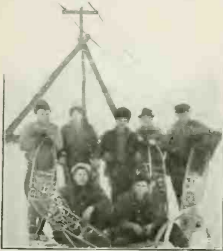
Instead of Spurs These Telegraph Linemen of Alaska Wear Snow-Shoes. The Poles Are Tripods Which Rest on the Ice and Snow.
