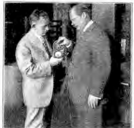
Fig. 6. Memory meter for depth sounding from aeroplanes which is part of the altimeter development of E. F. W. Alexanderson, consulting engineer of the General Electric Company. This memory meter intercepts the radio echo when it occurs, interprets it in altitude and preserves the result for observation by the pilot. Green, yellow and red lights give warnings corresponding to 250, 100 and 50 foot altitudes respectively. With Dr. Alexanderson in the picture is his assistant, S. P. Nixdorff at the left
