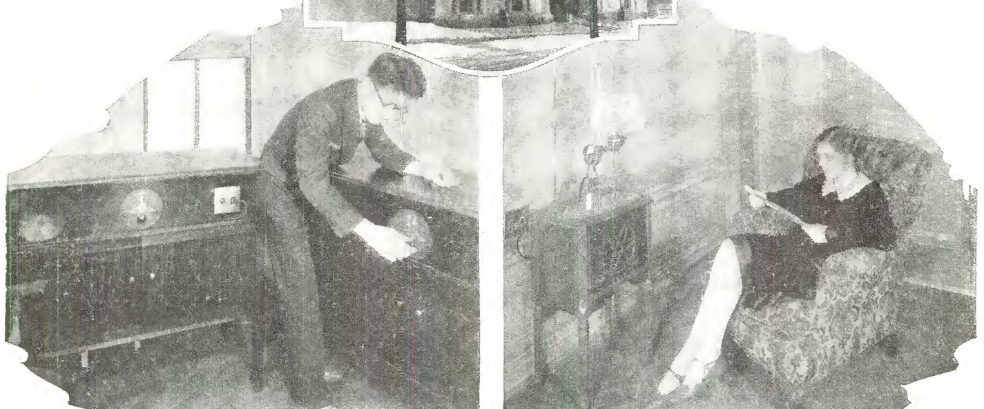
Fig. 1. This gives a composite idea of the Lake Lane Apartment installation described in the accompanying text. The upper photograph is the apartment building itself, the lower left shows the master receivers used in the radio room, while the lower right is the speaker installation in one of the 92 rooms that are so equipped in that building. The designer of the installation is shown in the lower left-hand photograph tuning one of the receivers
