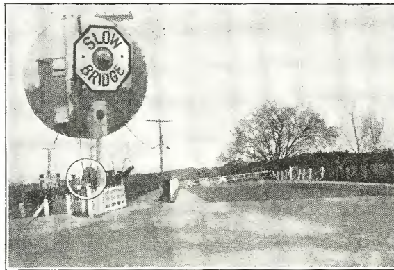
Fig. 8. Residents of Walpole, Mass., have noted the disappearance of certain raucous disturbances which were making radio reception in that vicinity unbearable. The mystery was solved when it was found that the stop blinker shown in the above photograph was causing the interference. The proper filter eliminated the disturbance
