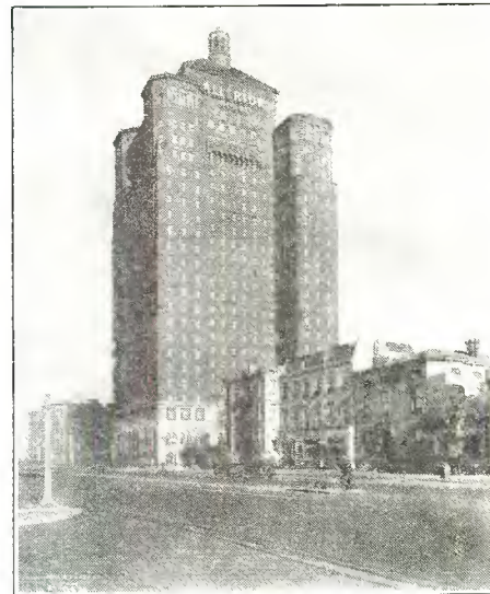
Fig. 7. The first major hotel installation of a centralized radio system was recently completed in the Allerton House of Chicago, the largest hotel of the Allerton chain
