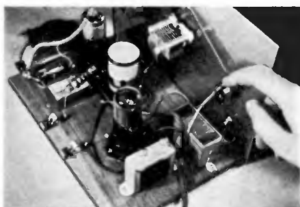
An S.P.S.T. rotary switch turns on the power
