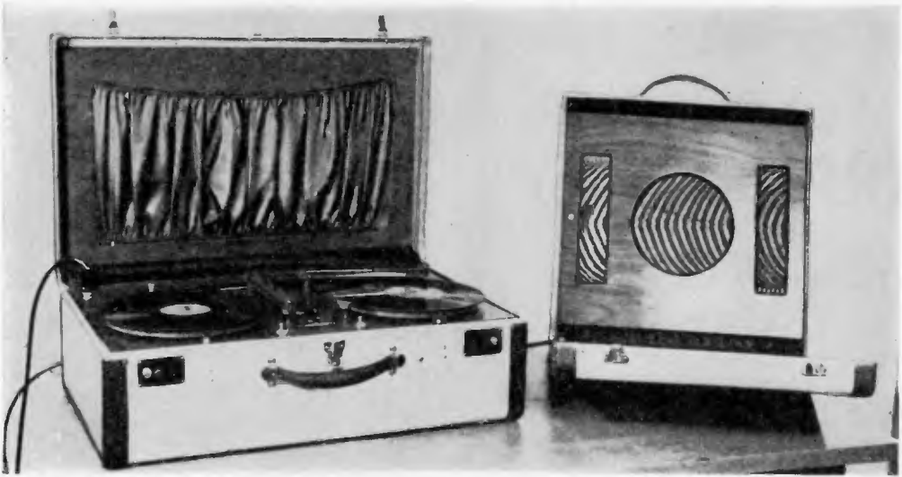
The twin phonographs and amplifier are installed in a 26" suitcase, the speaker in a matching hatbox
