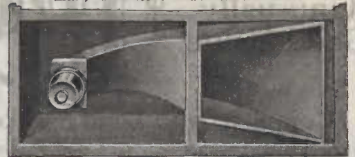
This View Shows the Interior Construction of the Loud Speaker Supplied with This Set
