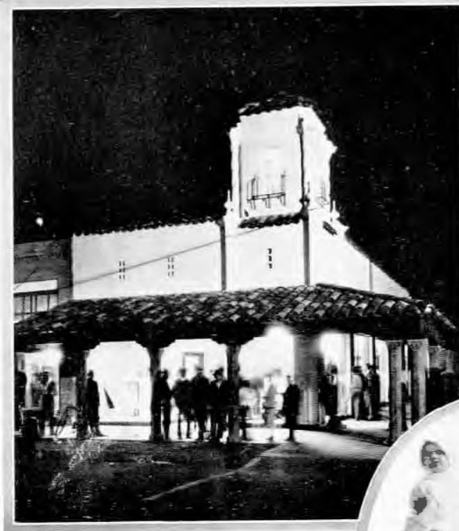
Thousands of citizens of Tempe, Arizona attended the opening of this new office of the Central Arizona Light and Power Company in that community. The town had previously been served by a municipal system.
