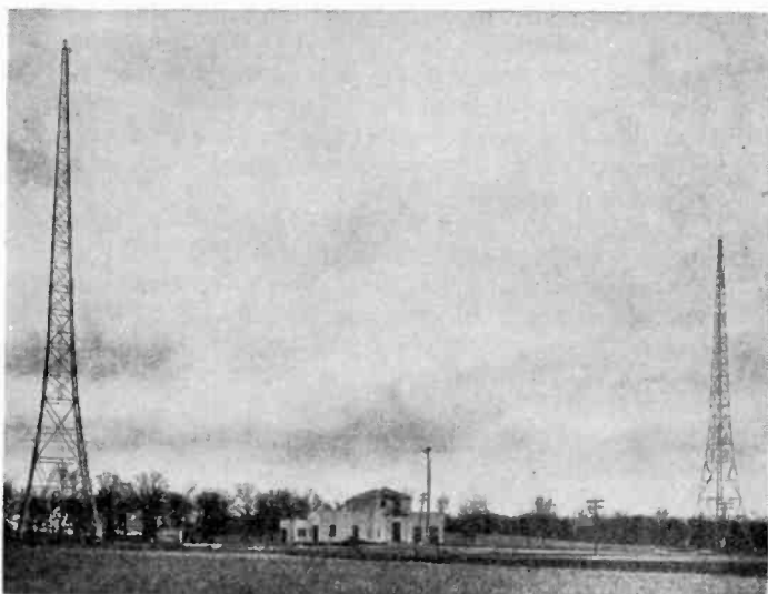
The hopping-off place. Programs are carried by wire from the studio in Chicago to the transmitter in the Spanish bungalow near Elgin. The steel towers, which support the antenna rigging, are 250 feet high.
