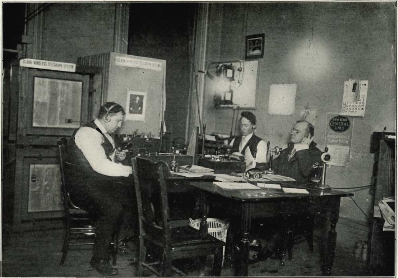
OPERATING ROOM, BAY CITY, MICH., STATION
