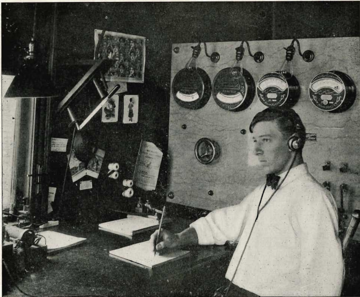
Clark Wireless Telegraph Station, Port Huron, Mich. Capacity 10 K. W. Thousands of vessel passages have been reported by this station. It is in daily communication with Buffalo, N. Y., 200 miles overland
