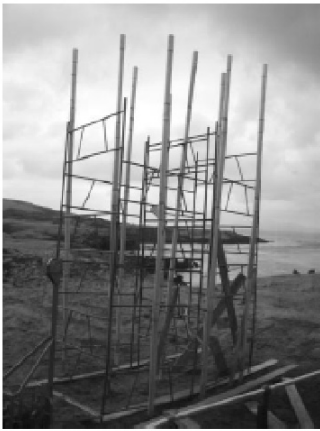
Fig 5: Erection of 15m antenna tower on Marion Island. Pictures courtesy of Pierre Tromp, ZS8M / ZS1HF.
