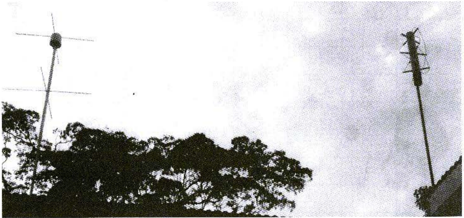
Fig. 4 Both antennae ready for reception on roof
