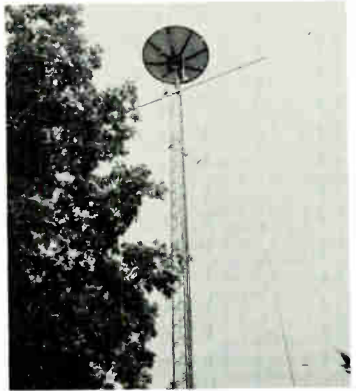
Figure 5. Dish is Parked Straight Up
