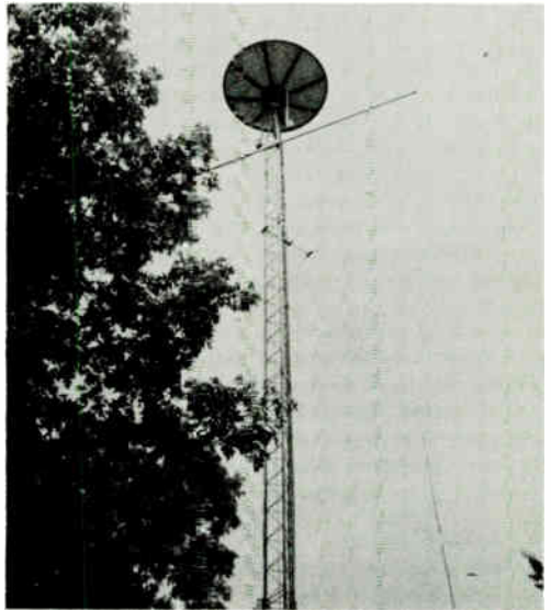
Figure 5. Dish is Parked Straight Up
