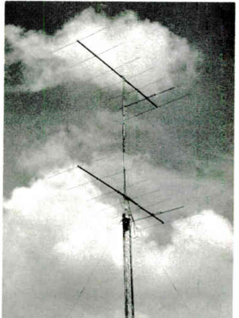
Vertically stacked 7 over 7 presently in use at WOBBM, pending completion of a more elaborate dual diversity array. Boom lengths 20 feet, vertical spacing 18 feet. Top antenna 80 feet above ground.
