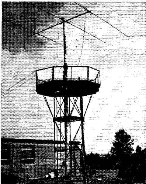
This photograph shows a practical application for a little-used war surplus item. The antenna belongs to WA9DZL, the ground communications section of the Wisconsin Air National Guard at General Mitchell Field, Milwaukee, Wisc. The antenna is mounted on a war surplus boom from a KC-97 mid-air refueling airplane. The beam is 27 feet high and can be raised hydraulically to 47 feet.
