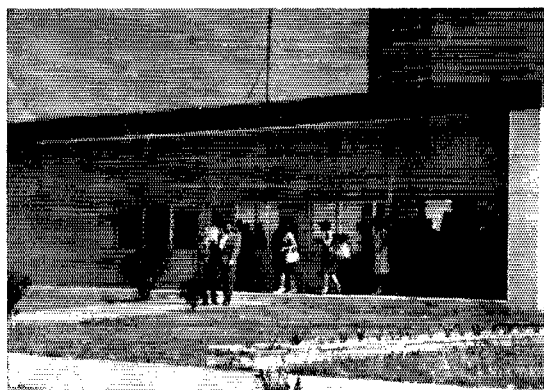
The new headquarters building of the Radio Club Dominicano. The tower, partially visible in the photograph, supports Vee beams on 80 and 40 meters. The club station call is H18RCD.
