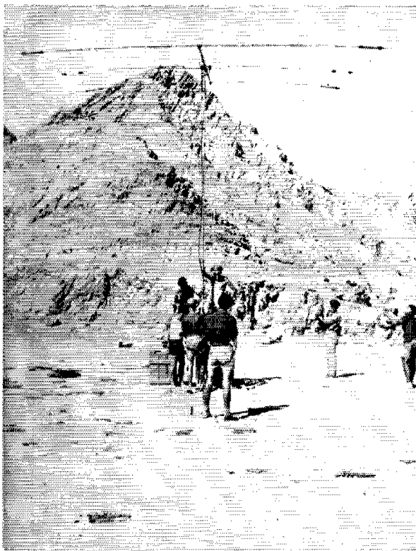
(Below) Putting up the TA-33 Jr. The mast would bend or break if we were not very careful!
