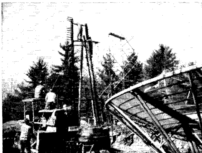
Work advancing slowly on the mount for the new dish at W1BU
