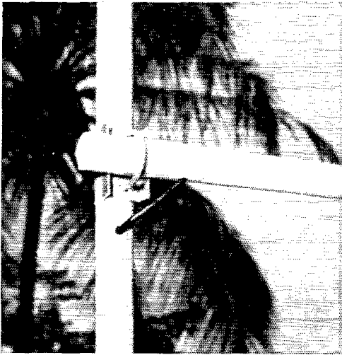
The booms are attached to the mast by means of TV U bolts and saddles. This view shows the coax line emerging from the upper boom and entering the top end of the mast. This and other detail views were taken with the crank-over tower in lowered position.
