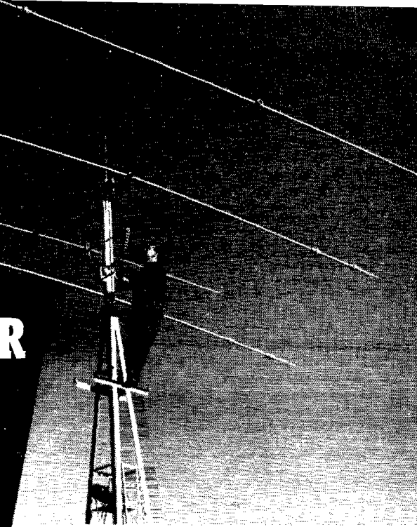
Vesto 60-ft. Tower supporting Telrex Model TBS-416 Beam and Model 175-R.I.S. Rotator.
