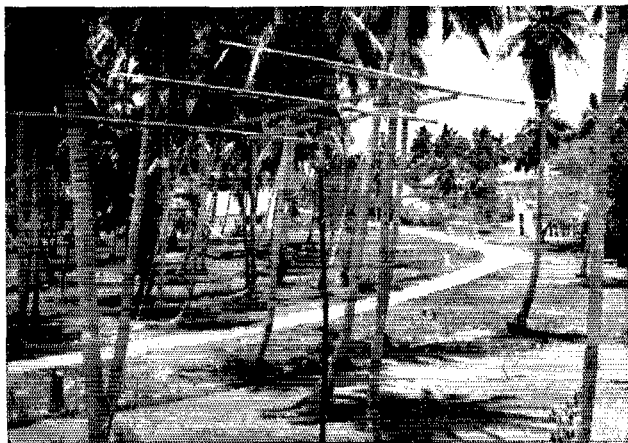
The beam was erected in the midst of some palm trees and was rotated by hand as the occasion demanded. Even though somewhat overshadowed by these trees, the signal was well received around the world.
