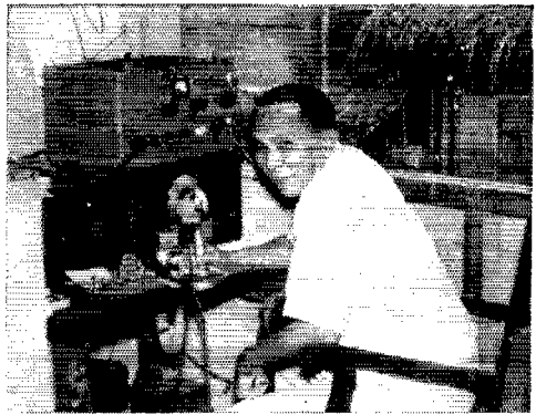
Du6IV is a familiar phone entry from Iloilo on 20, 15 and 10 meters. Mike's 1625 final is modulated by 807s and his hearing-aid is a modified HRO. (Photo via DUICE)
