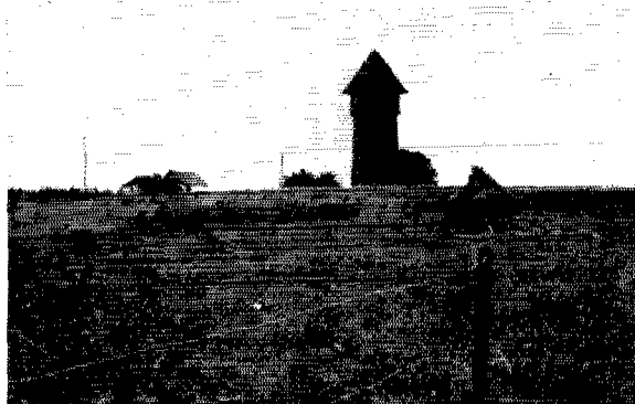
◆ Le chateau d'eau, as seen from a southeasterly direction. ◆
