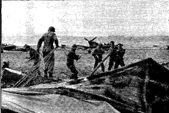
Signal Corps troops set up a mobile message center at an airdrome in North Africa. Top — Members of an aviation engineers unit dig a canvas-walled shelter for the SCR-299 near Youka les Bains in Algeria. Center — The radio truck is driven into its shelter and camouflage netting drawn over the top. Above — Additional camouflage completes the job. Right — Mobile signal battalion message center in Tunisia.
