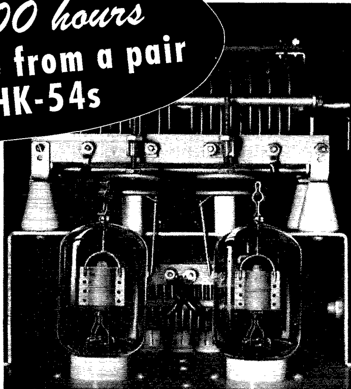
FINAL AMPLIFIER of the main station (WRAQ) at the Barnstable County Jail and House of Correction, showing the pair of Gammatrons still on the job after approximately 38,000 hours of operation.
