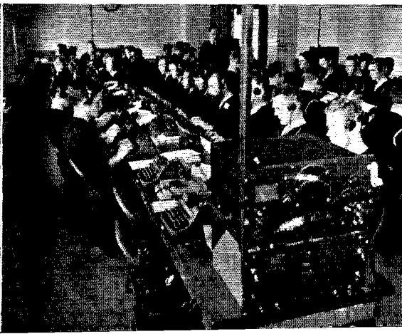
Left — Procedure class. Here the students learn how to handle traffic and carry on contacts the Navy way. Right — In the watch-standing room trainees gain experience in off-the-air copying of actual transmissions. Each table has its own receiver array as shown in the foreground, covering all Coast Guard frequencies.
