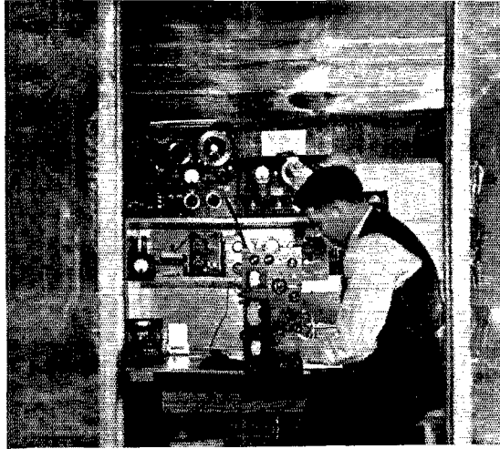
Shielded test booths are an important part of a modern radio plant. Outside QRN cannot be tolerated while critical adjustments are being made. Grounded copper screen completely encloses each test room.
