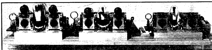
THE OSCILLATOR-AMPLIFIER 56-MC. TRANSMITTER AT W1HUV
