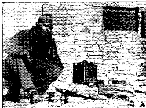
THE 5-METER EQUIPMENT TOGETHER WITH EXTRA RIBBON BATTERIES AND NUMEROUS FLASH LIGHTS AS USED ON THE ICE INSIDE OF THE CABIN
