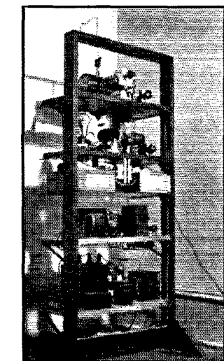
BREADBOARD TRANSMITTER UNITS REST ON THE BRACKETS PROJECTING FROM THE UPRIGHTS
