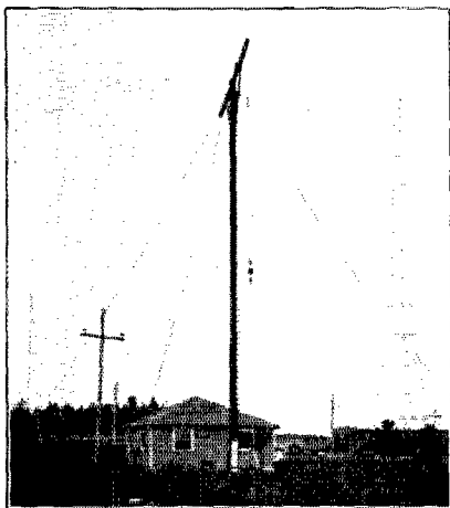
THE VERTICAL HERTZIAN ANTENNA AT 2XAF.
