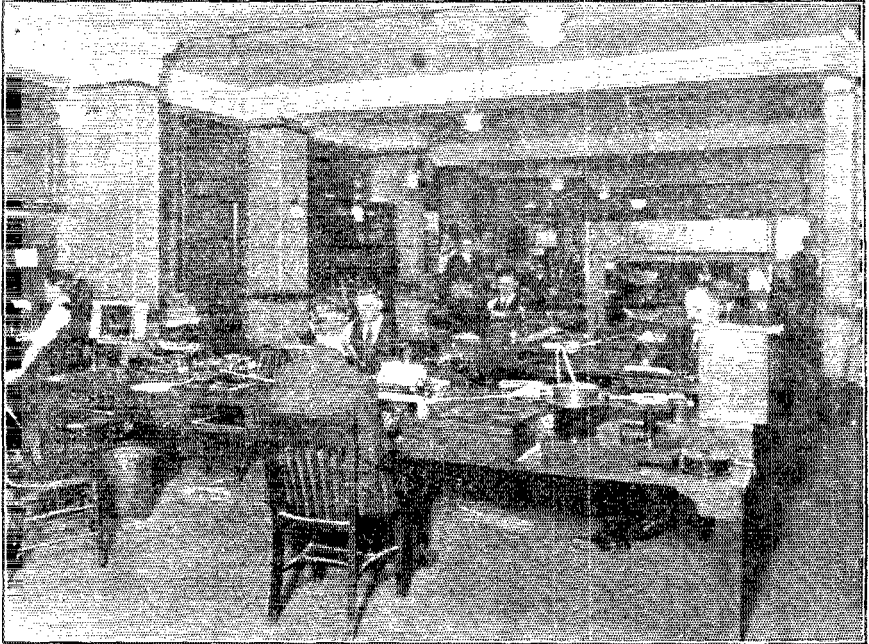
Above: Main Operating Room at New York.
