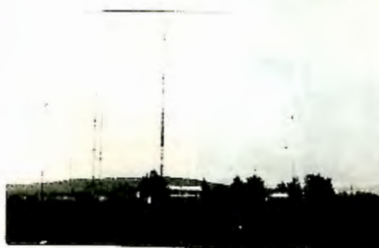
The transmitter site at Holzkirchen. The two nearest masts are part of the MW antenna array. A dipole array for SW can be seen in the rear of the transmitter house. The foothills of the Alps are just visible in the background.
