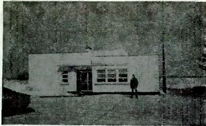
CHU transmitter building with Hamilton in front.
