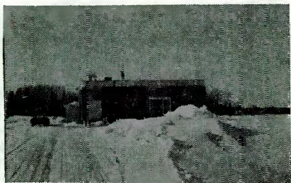
Stanley Corners Monitoring Station from the driveway.
