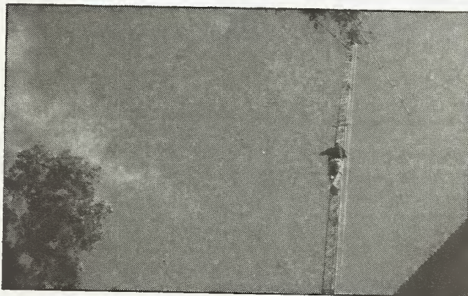
Scotty, W7SW/VK9YT, climbing the 70 foot tower to make adjustments to the log-periodic antenna on Home Island in the Cocos Keeling group.
