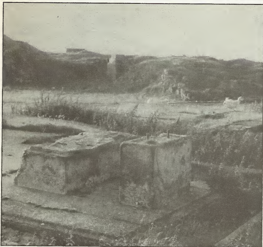
View to the NW showing the original aerial mount in the foreground.
