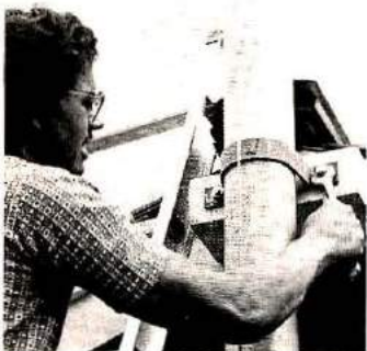
Mounting the House Bracket
