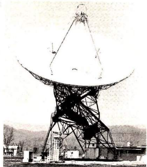
A closer look at one of the 85-foot antennas. This is the Howard E. Tatel telescope, one of the oldest at the observatory. It is the fixed part of the interferometer array; the other two are movable along a track in order to obtain a variable baseline ( photo courtesy NRAO ).
