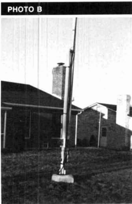
PHOTO B Base of W4OTS tower. Tower is affixed to ground post sunk in cement. Clevis at top of post permits to tilt over. The mast is locked in position by second clevis near base of the ground post.
