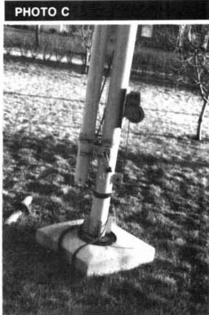
PHOTO C Closeup of ground post and base of mast. Winch is mounted to side of post. Tower was designed following data provided by Bob Haviland, W4MB.
