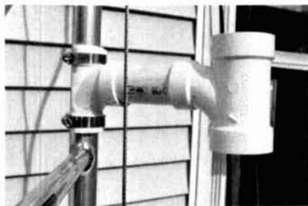
One of the cable guides installed on my tower.
