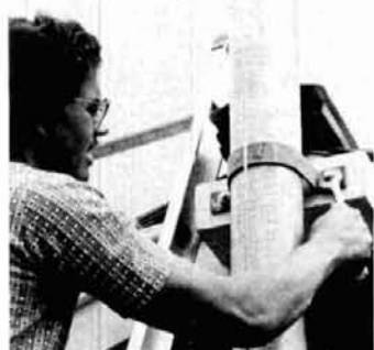
Mounting the House Bracket
