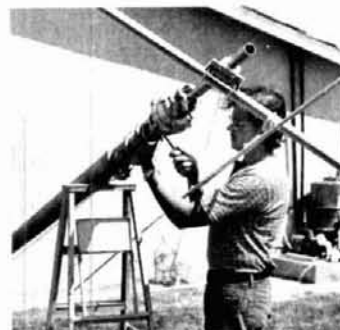
The Hinged Base Plate allows tower to be tilted over for access to antenna and rotor from the ground.
