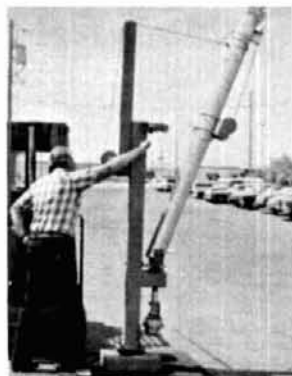
Tilting the tower over is a one-man task with the Wilson bases.
