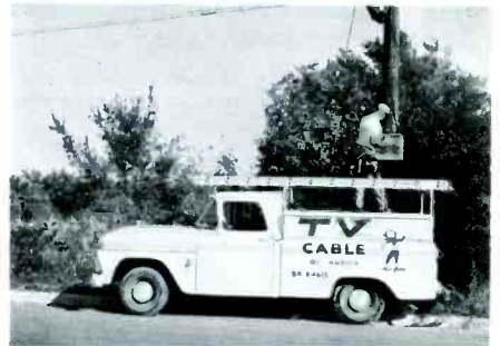
TV Cable technicians install amplifier, operating from radio-equipped service truck.
