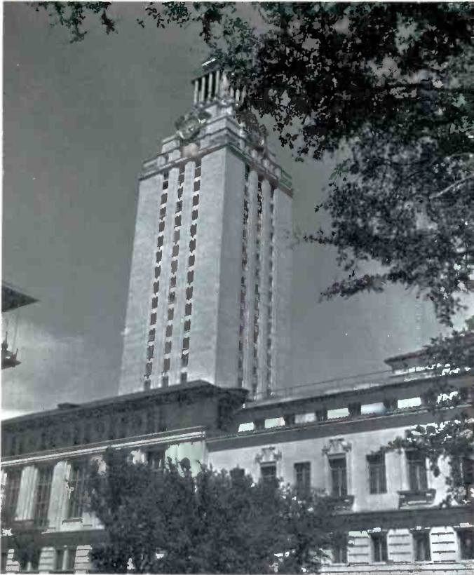
The University of Texas Tower (main building) houses a million volume library. On the 27th floor is microwave equipment for TEMP. Sheets of plastic (see center windows, 4th from top) on the south and west sides replace regular windows with bars to permit better transmission through a non-metallic material.
