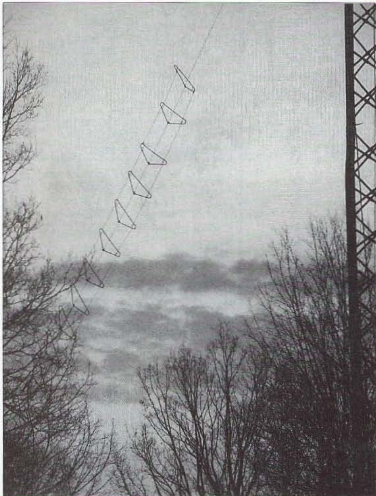
Photo B. Upper half of WARC dipole with lower half blending into the landscape.
