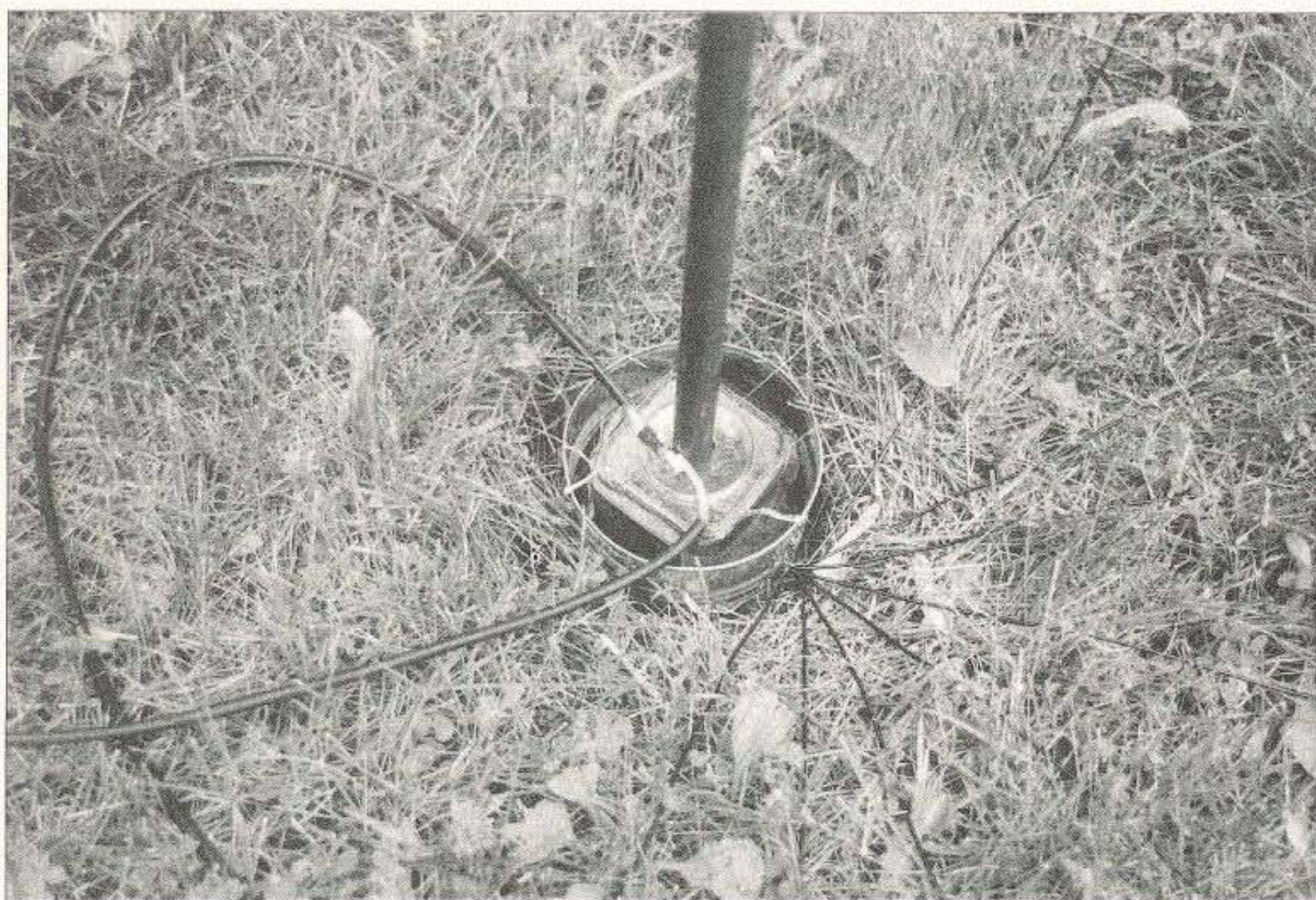
Photo B. Each antenna is supported on a glass insulator which is an inverted glass jar partially sunk into the ground. The 296 ml (10 oz.) jam jar shown here has a concave bottom that helps keep the antenna in place. The jar fits inside a 796 g (28 oz.) tin can which is sunk into the ground. The can holds the glass jar in place and provides an initial grounding point for the coax and the antenna. Radial wires are connected to the can.
