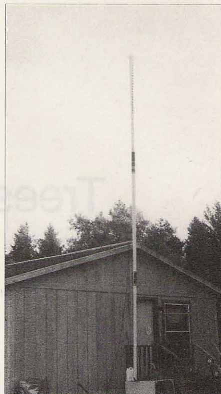
Photo C. The three-inch by 30-foot mast at work.
