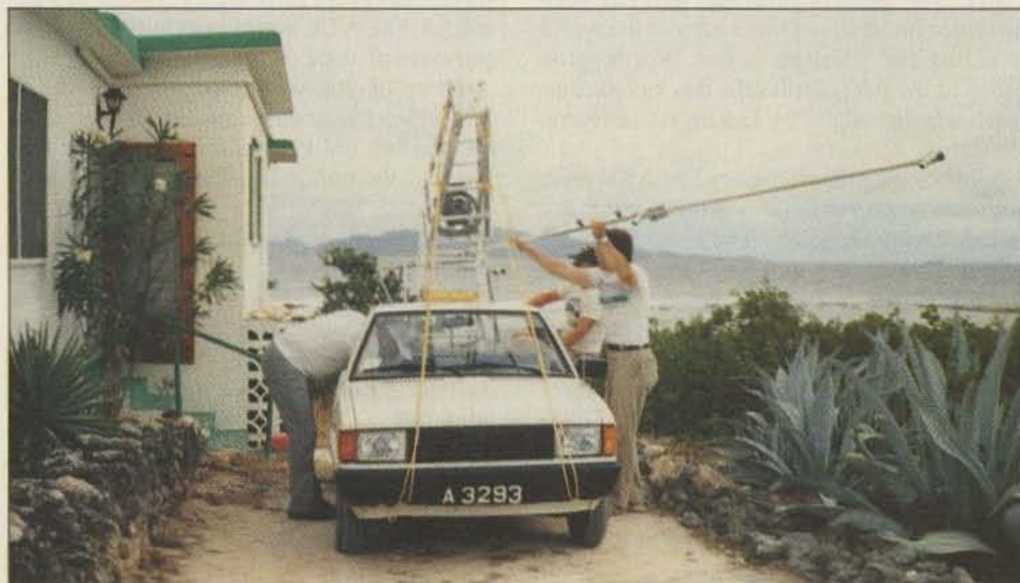
Photo B. The tower for VP2EOH was borrowed from an Anguilla ham, and the tribander was donated to the island's Boy Scouts afterwards.
