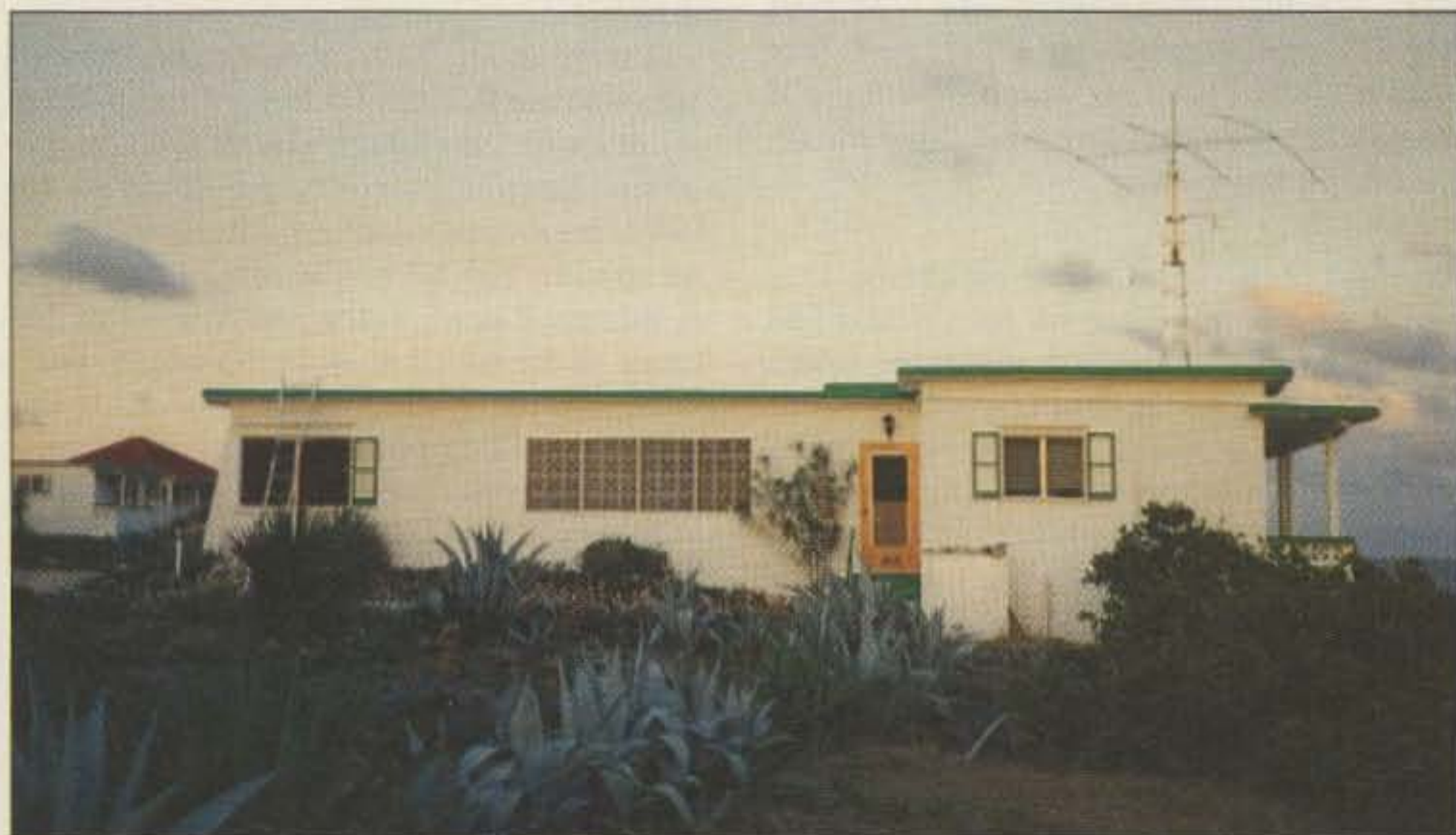
Photo A. The VP2EOH DXpedition's main operating location—a seaside villa on Anguilla. Note the 15-foot tower and tribander on the roof. The flat roof made antenna installation easy.
