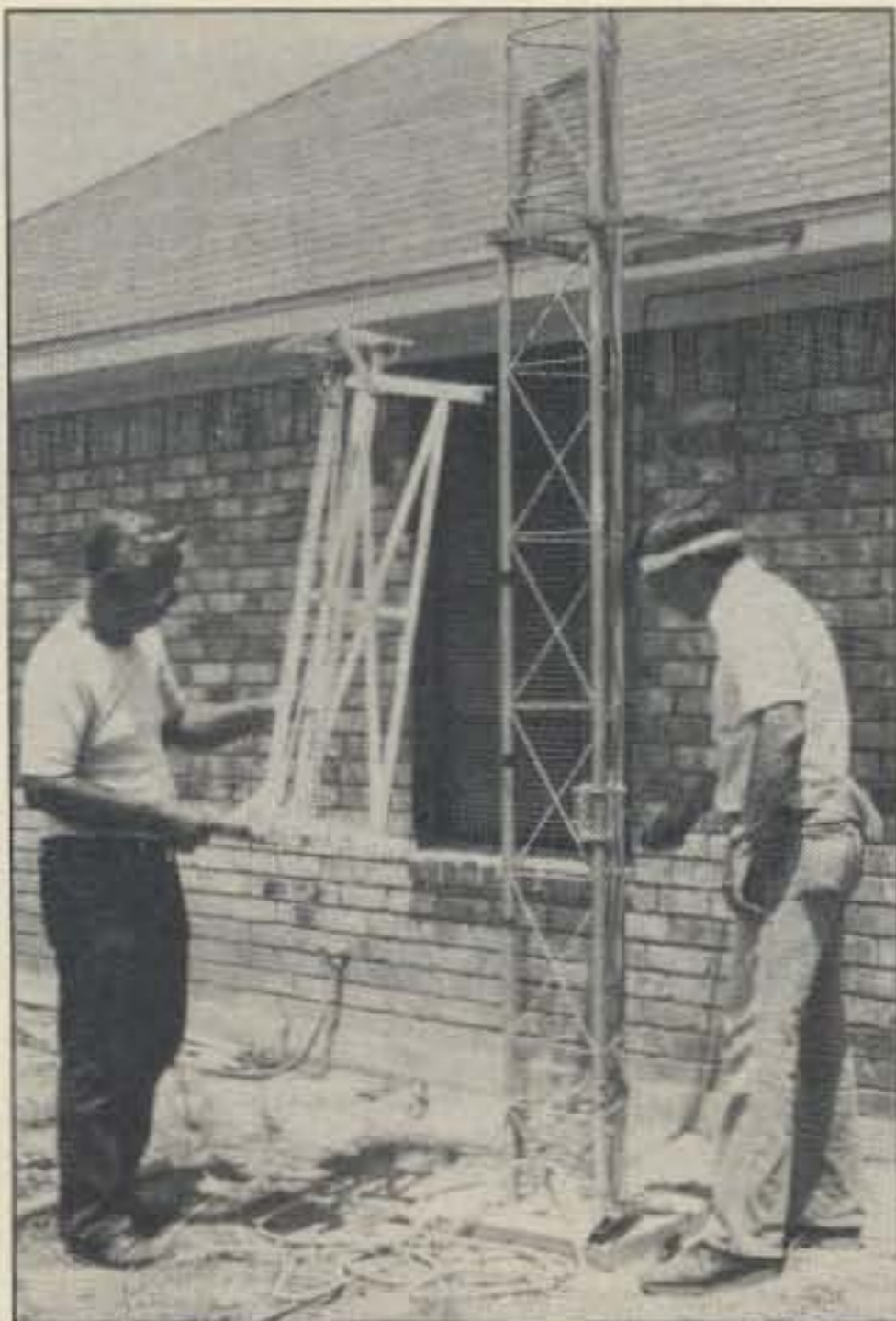
Photo C. Winching the the two Hazer side parts above the house bracket.
