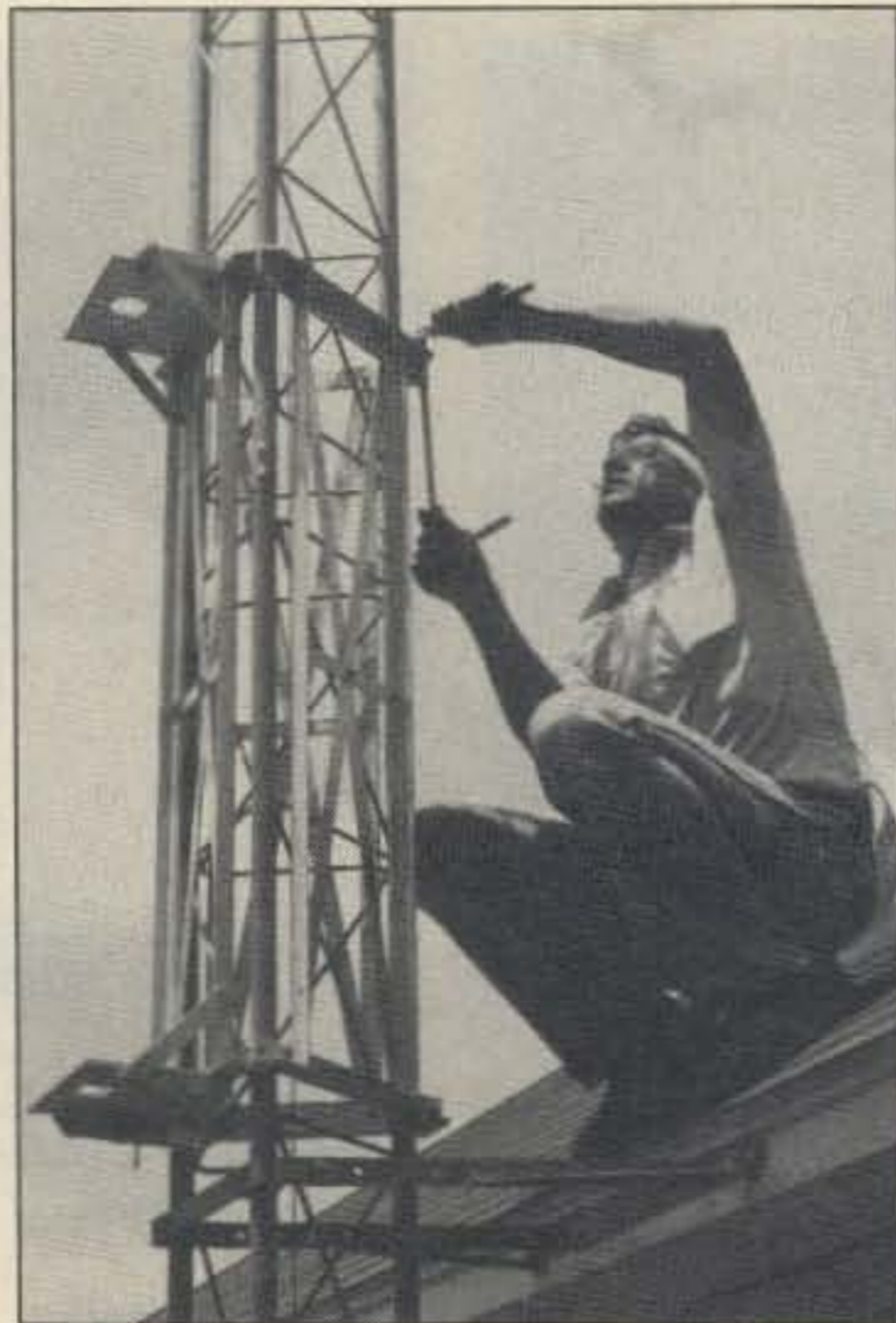
Photo D. Final bolt tightening before antenna installation and raising.
