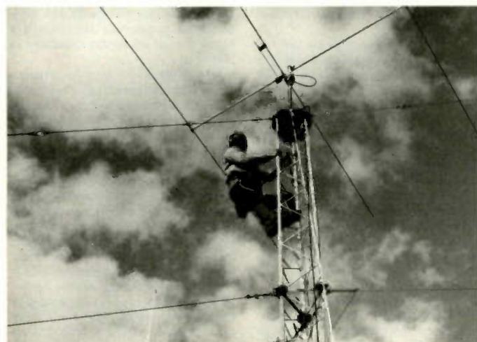
5B4CV doing some antenna work.
