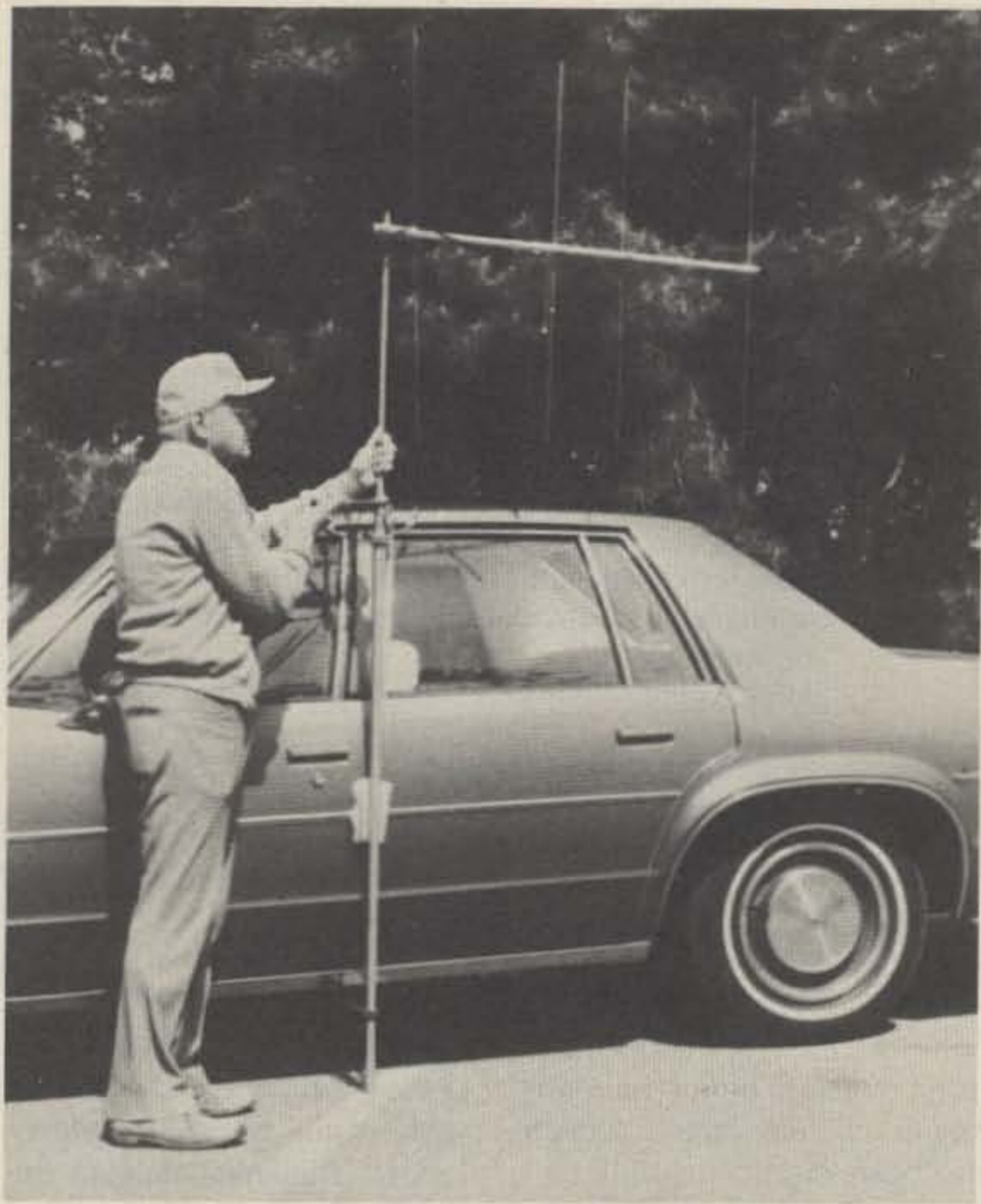
Photo C. Beam and transmission line installed; mast being extended.
