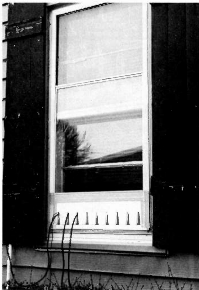
Lines in; window weatherproofed.
