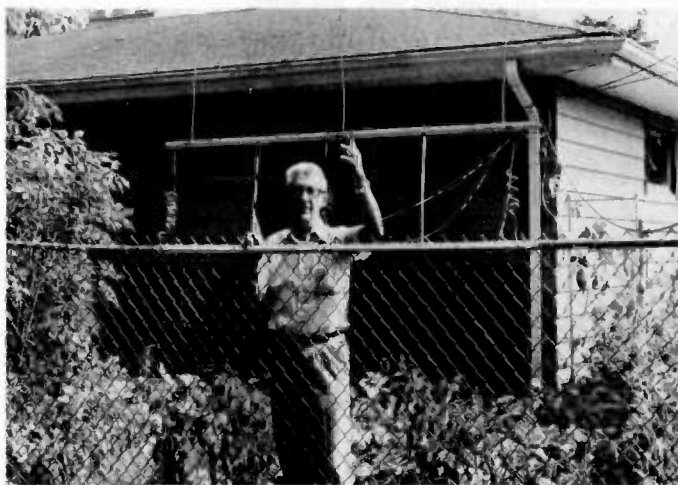
Photo A. Because trees bow and curtsy in the wind, and because vertical wires suspended from them thus dance up and down, some sort of flexible bottom-end tie-down is needed if an antenna orchard is to survive heavy gusts. I devised a "sway bar" system to beat the wind. Here, I'm checking its position. It's a five-foot fiberglass fence post tied with two screen-door springs to another such post strapped to the top pipe of a chain-link fence. The springs stretch and contract in the wind, maintaining tension on the vertical wires. The spiral pigtailed wound into the antenna elements allow them to flex as the sway bar moves up and down.
