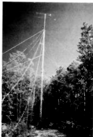
Photo A. Ropes are run to the top of the tower for hoisting the antenna. (Photos by Cindy Brown)
